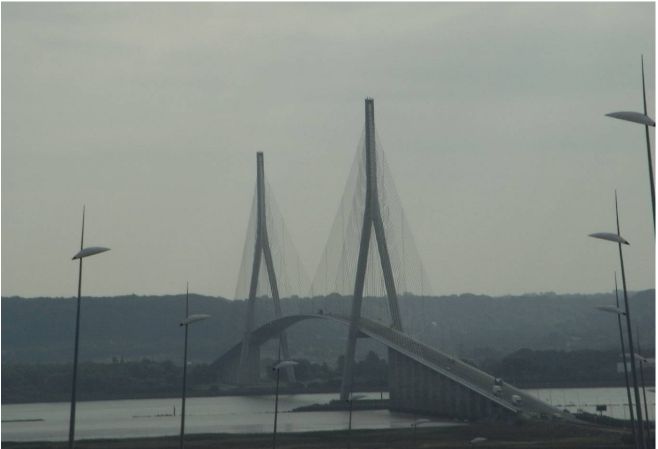
The Normandy Bridge
